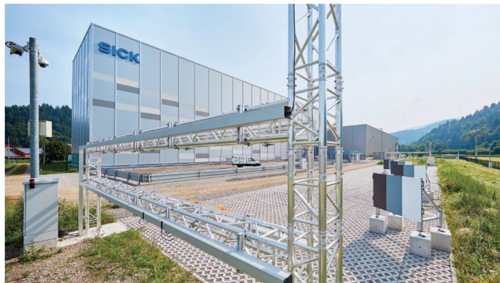
SICK’s Outdoor Technology Centre (OTC)
