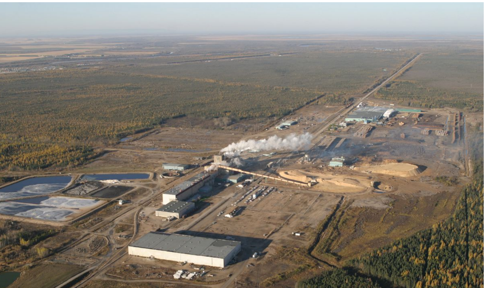
A former Tolko mill and its site in The Pas, Manitoba became Canadian Kraft Paper after being purchased by the AIAC in late 2016.
